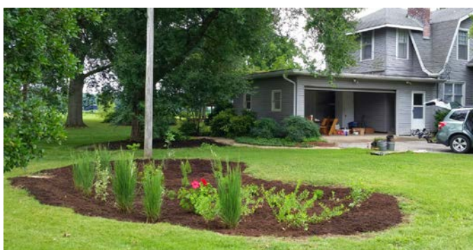
A rain garden catches rooftop and driveway runoff at UT's West Tennessee AgResearch and Education Center in Jackson, Tennessee.
