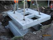
STREETS—Paving of Six Streets—Before the milling and paving can begin, the contractor was required to make repairs to the culvert on Chickering Lane by replacing the existing deteriorated corrugated pipe with concrete pipe and installing a new storm grate and stone headwalls. The work was just completed at the time of the newsletter publication, and the contractor plans to begin milling the streets before the end of the month.
