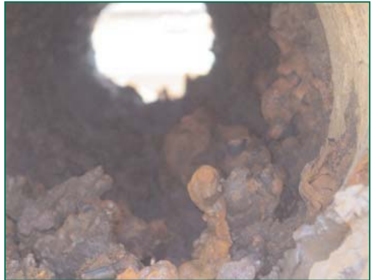
“Typical condition of water lines to be replaced.”
